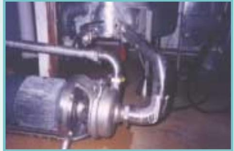
A complete overhaul - including rewinding the drive motor, replacing the motor bearings, checking and cleaning the pump bearings, and repacking the pump glands - reduced the noise by 27 dB(A).
